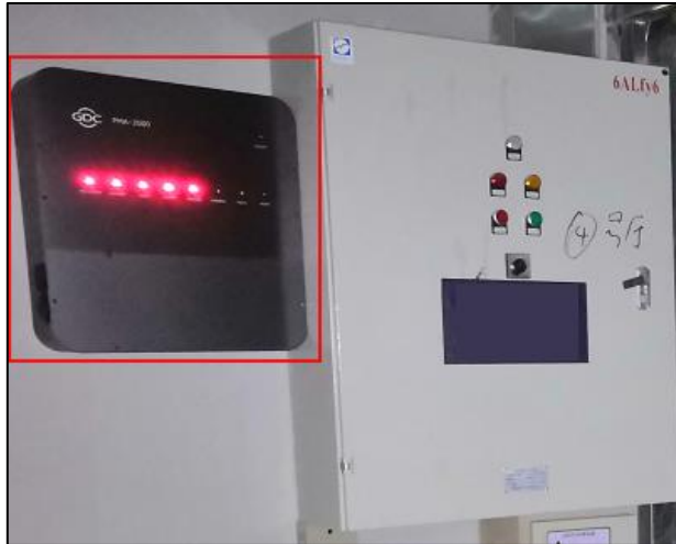
Figure 1: Mounting location for PMA-2000
