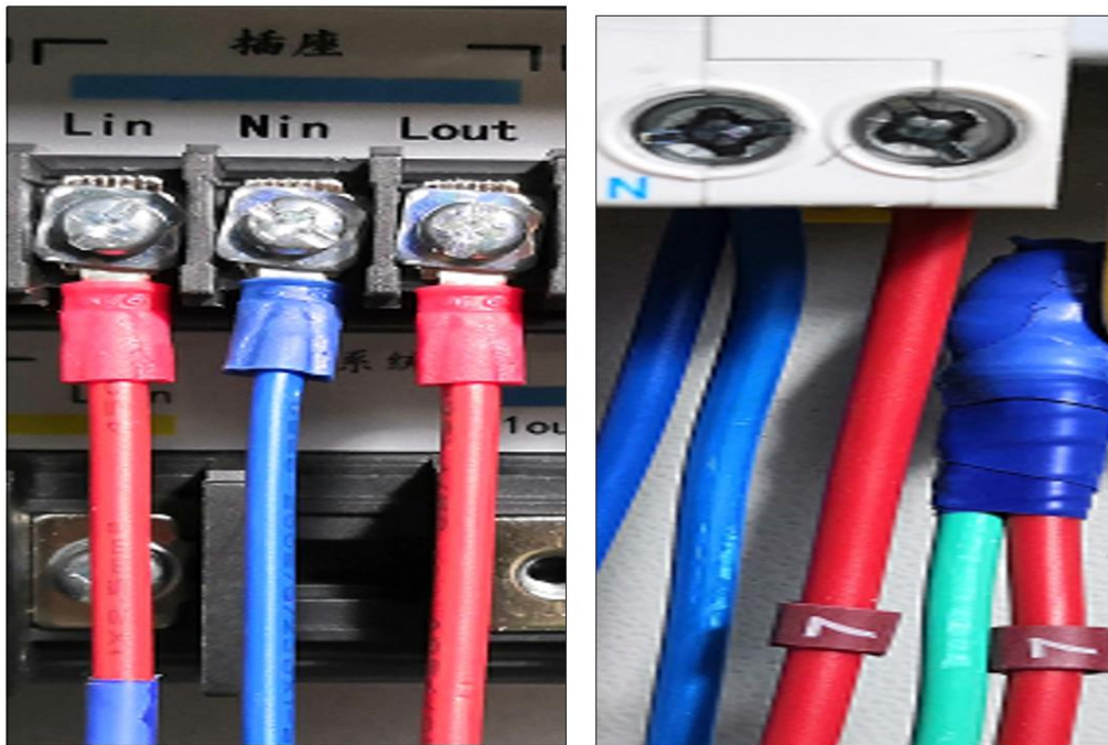
Figure 10: Device Socket circuit breaker connection
